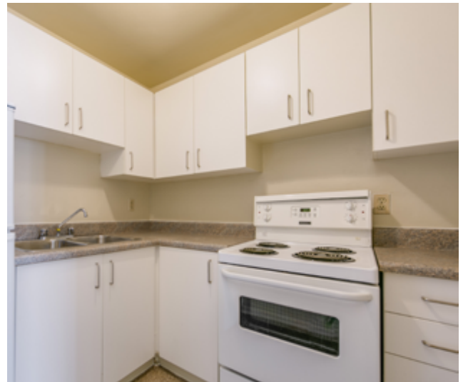
Charles Street kitchen before refurbishment.
